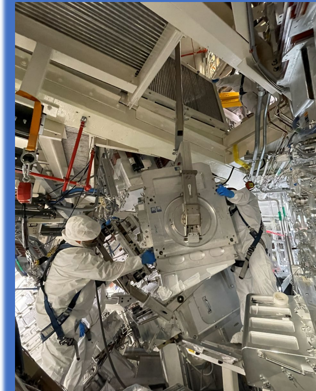
Hoisting & Rigging IOM into place
