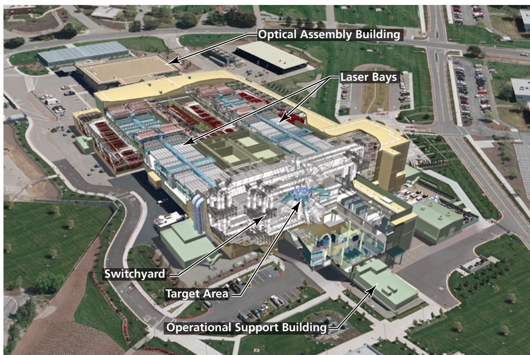
Figure 1-1. National Ignition Facility (NIF) aerial view, showing the two laser bays, switchyard, target chamber area, Operational Support Building, and Optics Assembly Building.
